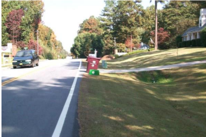
Figure 3.4 - Typical LID/GI practice: grass channels & rural section in place of concrete curb & gutter (3-5)
