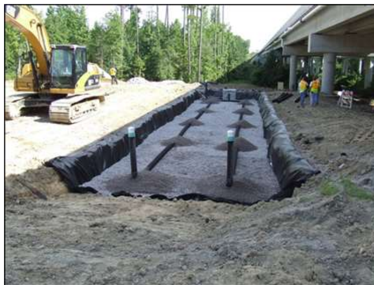
Figure 10.8-4 - Typical underdrain installation (photo courtesy of NCDOT)
