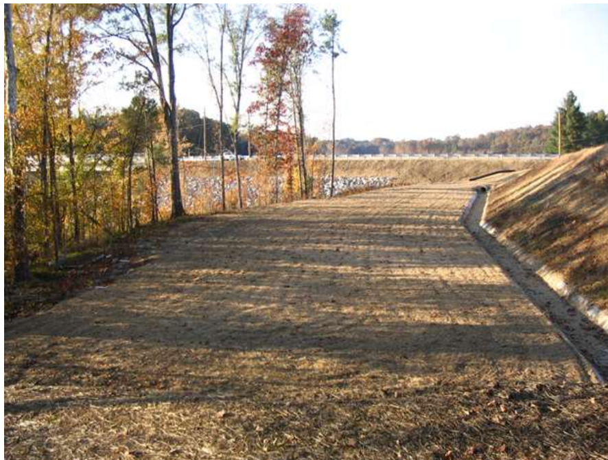
Figure 10.8-6 - Typical level spreader configuration (photo courtesy of NCDOT)
