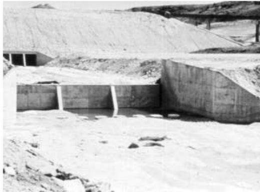
Figure 8.22 - Straight drop spillway stilling basin
