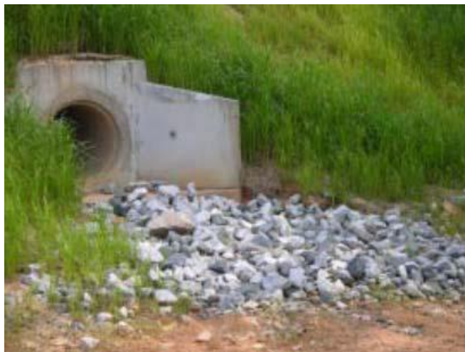
Figure 3.2 - Typical riprap energy dissipator (3-5)
