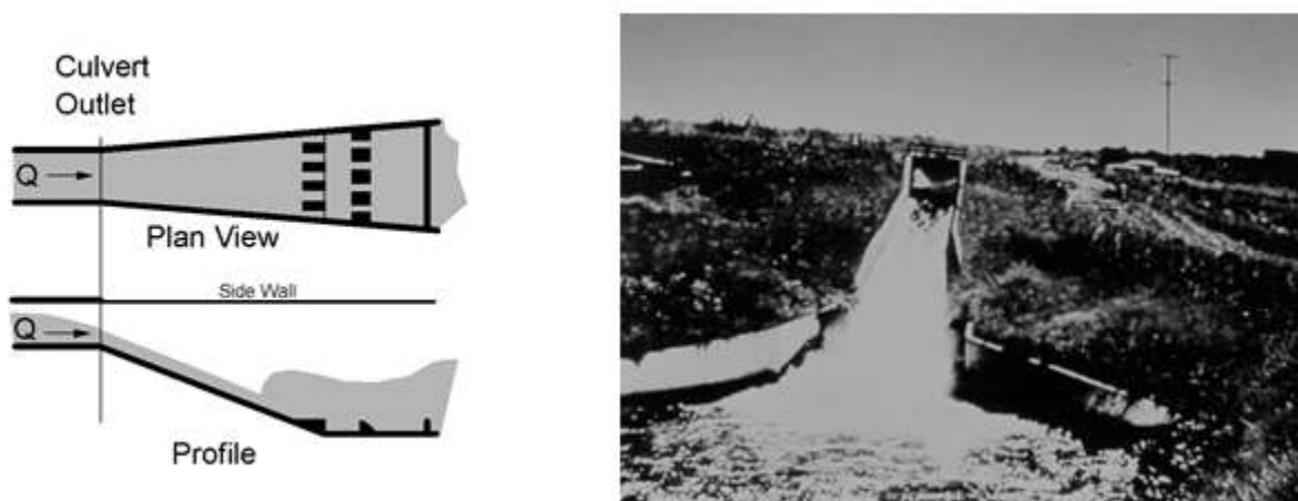
Figure 8.20b (right) - Photo of SAF stilling basin
