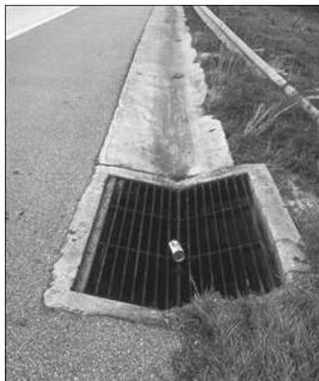
Figure 6.4 - Photograph of typical v-section gutter and inlet
