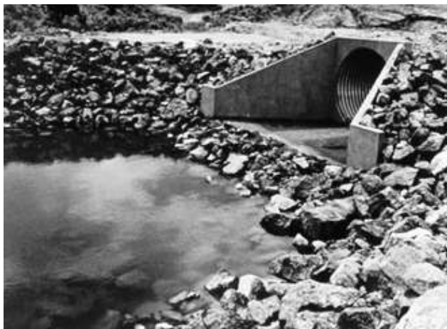
Figure 8.24 - Riprapped culvert energy basin
