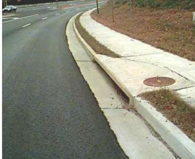
Figure 6.7 - Curb inlet placed on continuous roadway grade
