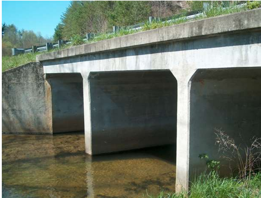
Photograph 8.2 - Embedded box culvert
