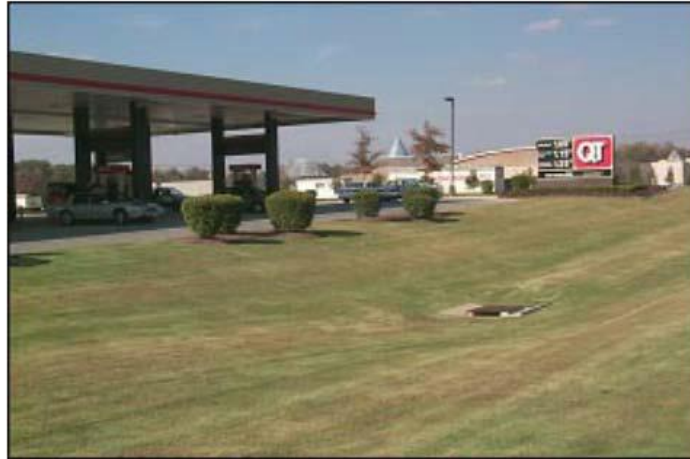
Figure 3.3 - Typical post-construction BMP - grass filter strip (3-5)
