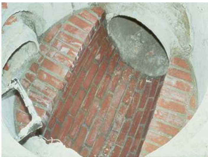
Figure 7.11 - Example of a bench in an access hole
