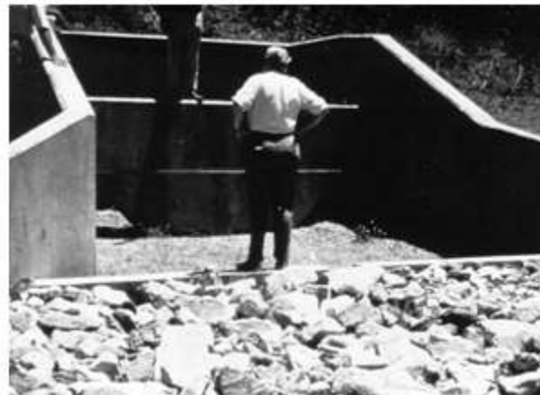
Figure 8.21b (right) - Photo of Baffle-wall energy dissipator - USBR Type VI
