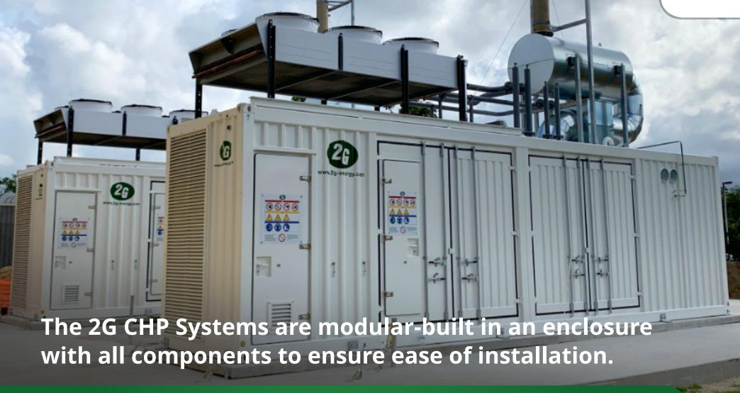
The systems are customized for RBF's specific project needs, delivered to the site fully tested and ready to connect to the corresponding electrical, mechanical, and communication points.
