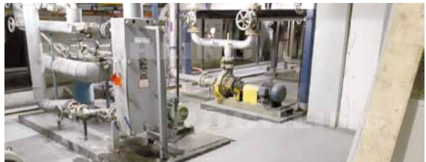
Foamlite® P cubic grain as a slip-resistant floor surface of a paint shop in the automotive industry
