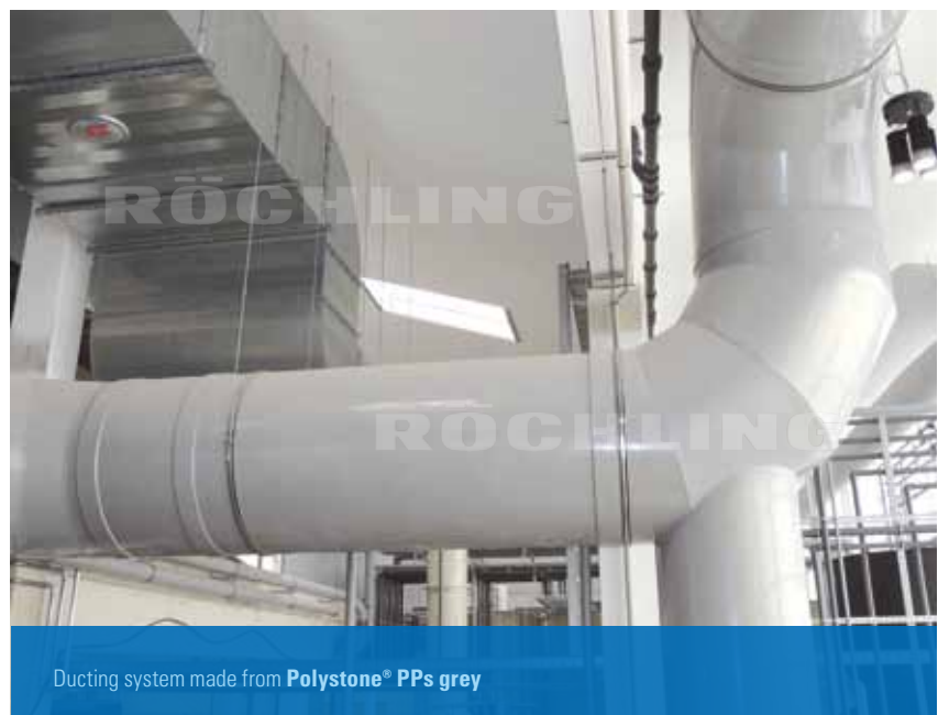
Polystone® P homopolymer grey Ventilation system for a galvanic plant
