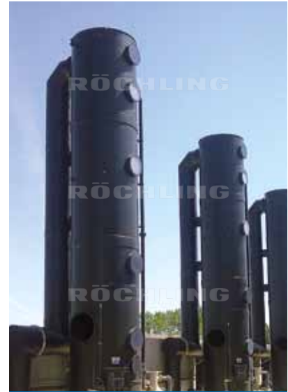
Polystone® G black B 100 exhaust air scrubbers of a domestic waste sorting plant
