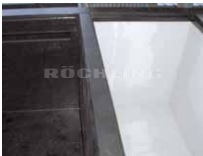
Polystone® PVDF GK Inliner of a chrom-plating bath
