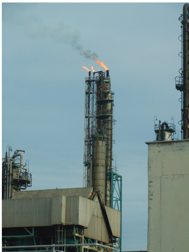
Figure 6. Flare before installation of FGRU.
