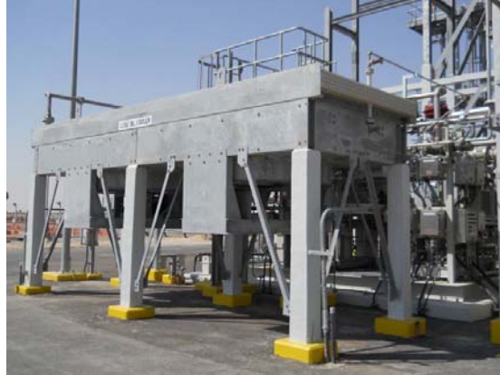
Figure 7. Air-Cooled Heat Exchanger for an FGRU System
