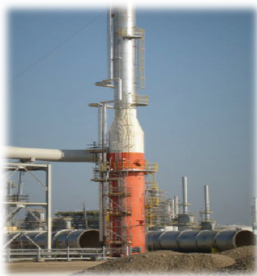
Figure 6. Deep Liquid Seal Drum for an FGRU System
