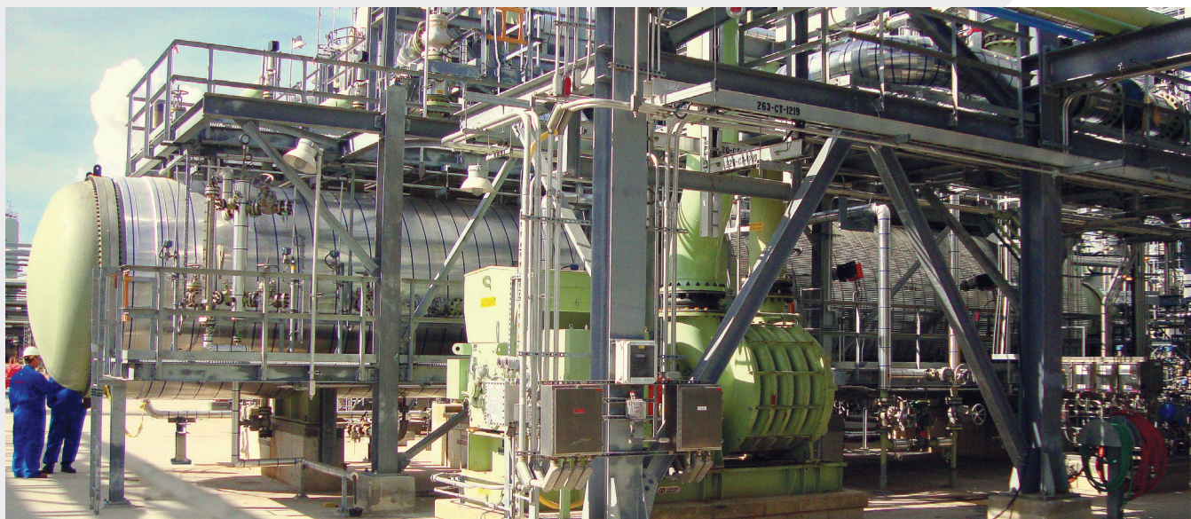
SRU reaction furnace with firetube waste heat boiler
