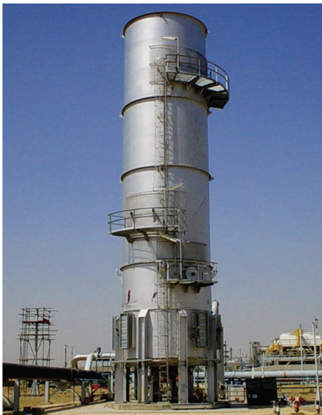
Natural draft SRU tail gas incinerator
