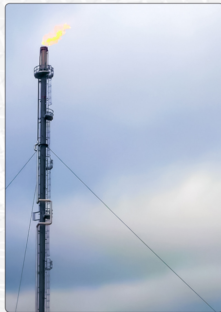
Proper application of steam allowing luminosity in the flame and full combustion
