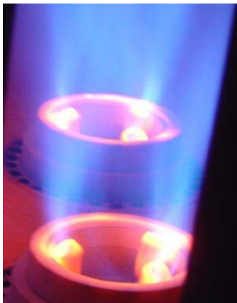
Valero St. Charles Refinery Freejet™ Installation
