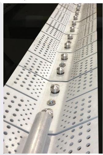
Low-NO<sub>X</sub> Duct Burner
