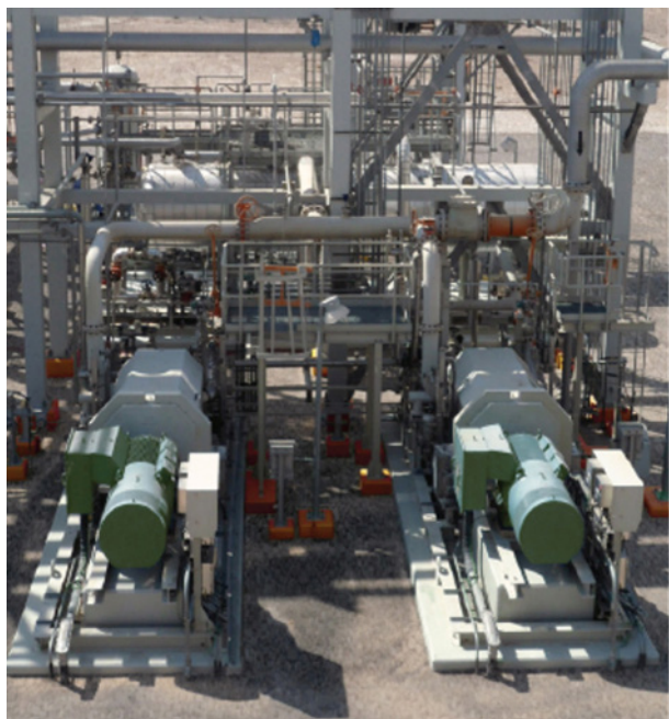
Figure 5. Zeeco FGRU system installed in a facility in the Middle East.
