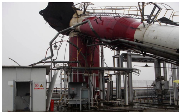
Figure 6. Destroyed flare stack as a result of flashback.
