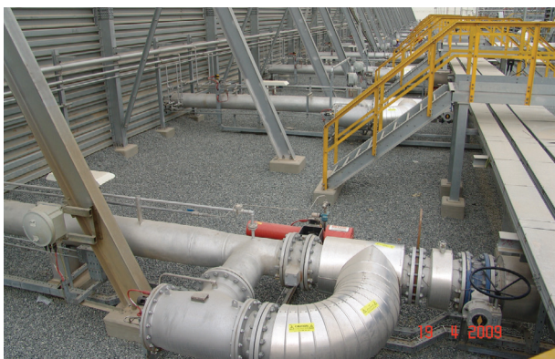
Figure 2. Typical installation of MPGF fence.
