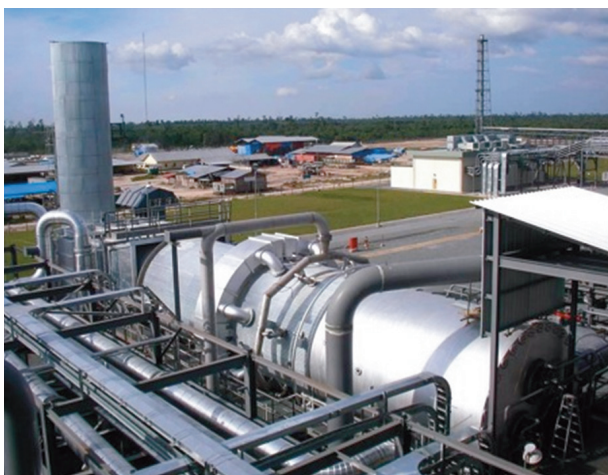
Figure 4. A permeate and acid gas thermal oxidiser with a hot oil heater.
