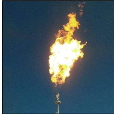
Figure 2 – Example of Sonic Process Flare
