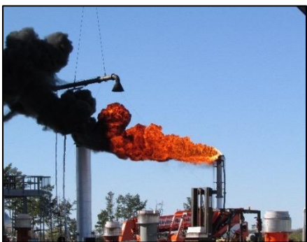
Figure 3c – Example of Smoking Flare System
