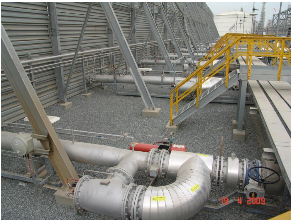
Figure 2 – Typical Installation of MPGF Fence
