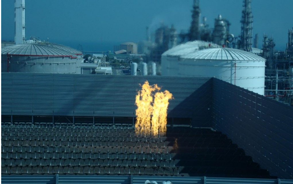
Figure 1 – Typical Installation of a MPGF
