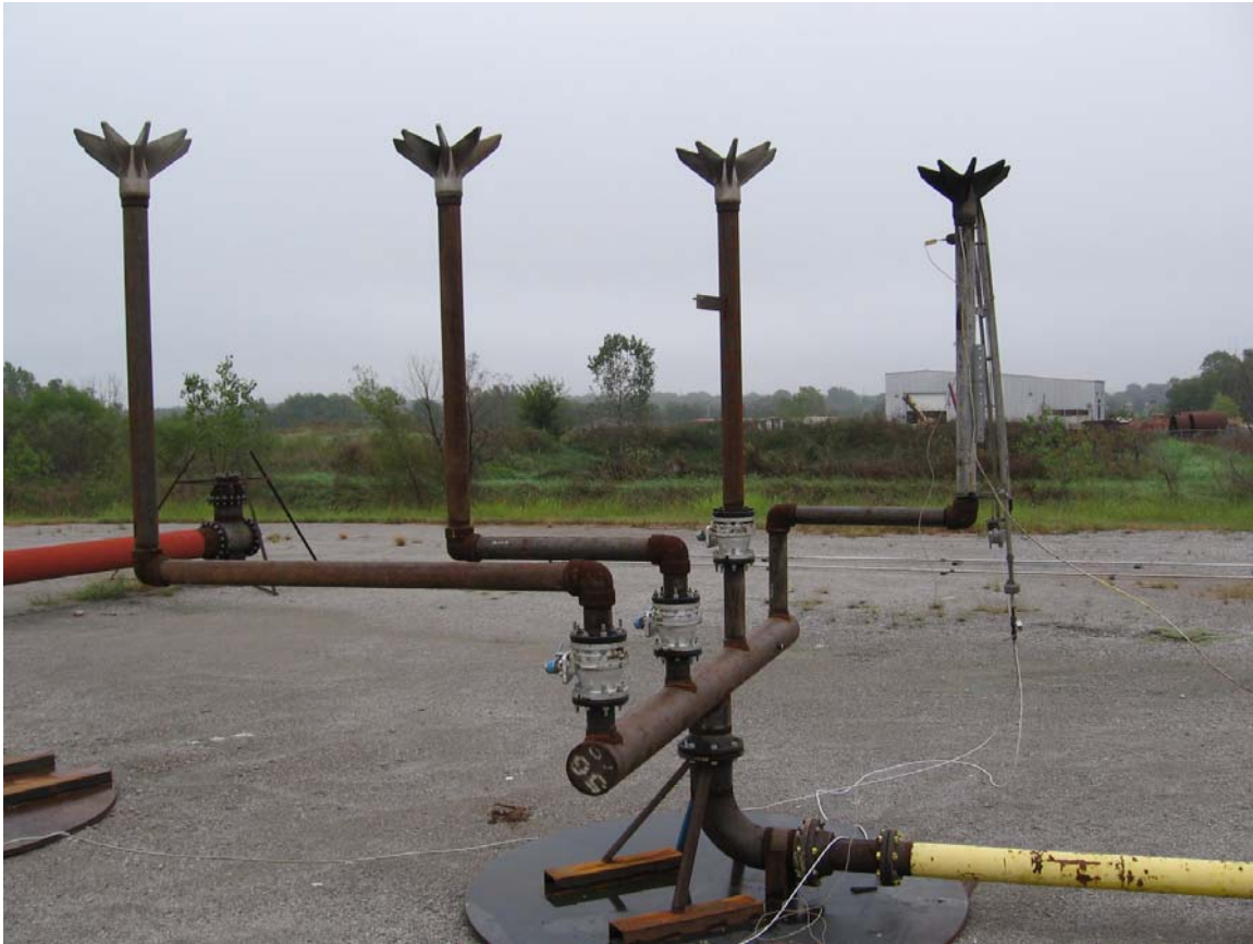
FIGURE 6: Flare Burner Test Pig
