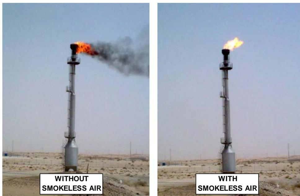
Figure 11. HPAAS flare system installed in the Southern Area
