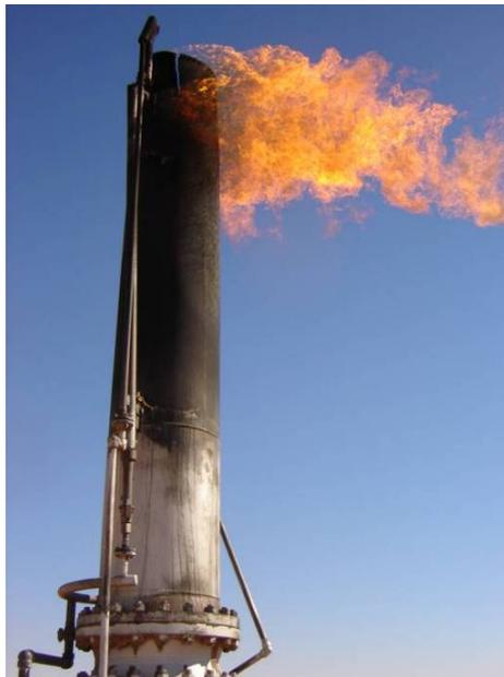
**Figure 2. Utility flare showing damage from flame pulldown**
