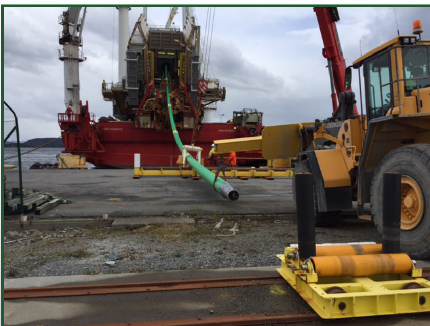
12" I-PEP installed in end of spool to allow reeling onto vessel
