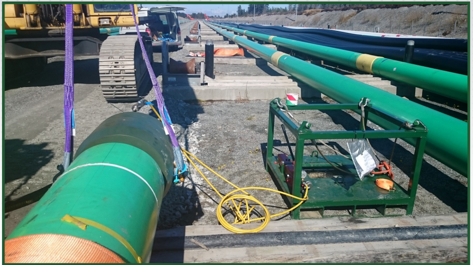
12" E-PEP installed to pipe spool
