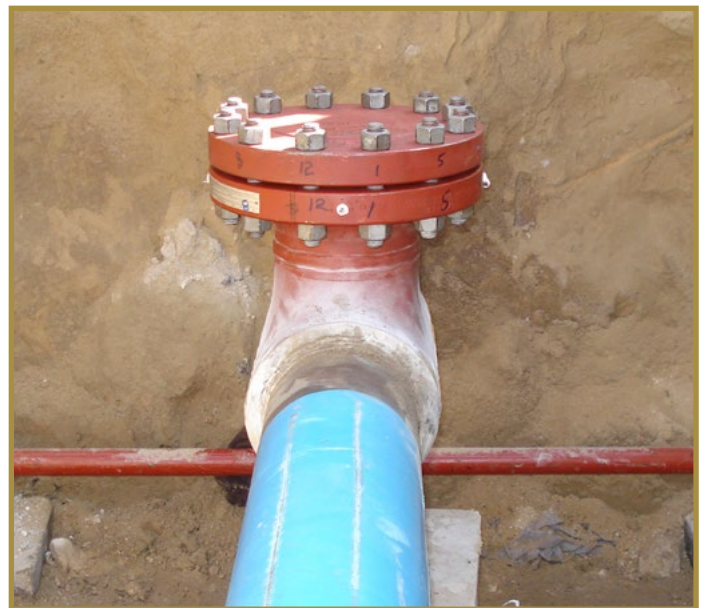
Completion plug and blind flange fitted to the split tee fitting
