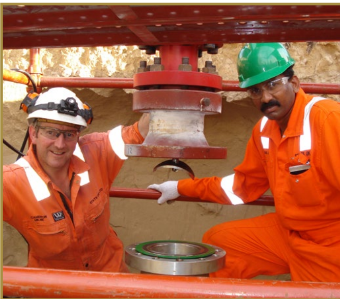
Hot tap machine and pipe coupon removed
