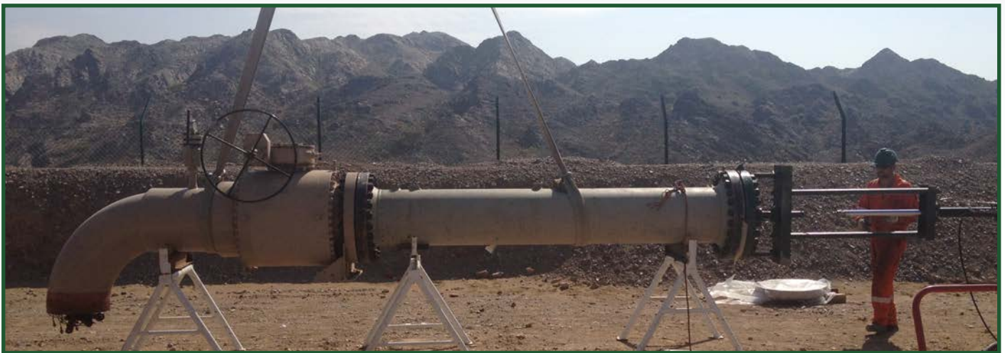
Bend, valve and deployment launcher removed
