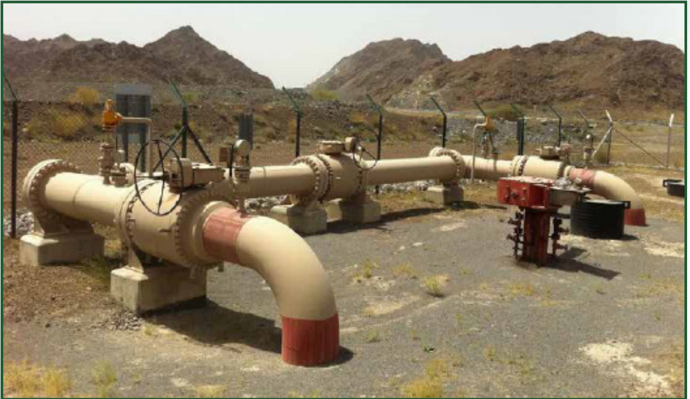
Block valve station (BVS) bypass pipework
