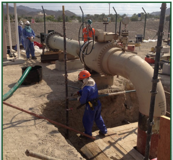
Tecno Plug™ deployment system housed in pressure competent launcher
