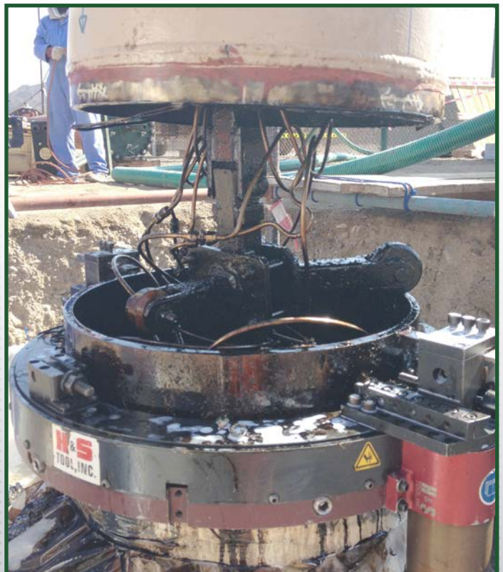
Pipework cut allowing bend, valve and launcher to be removed
