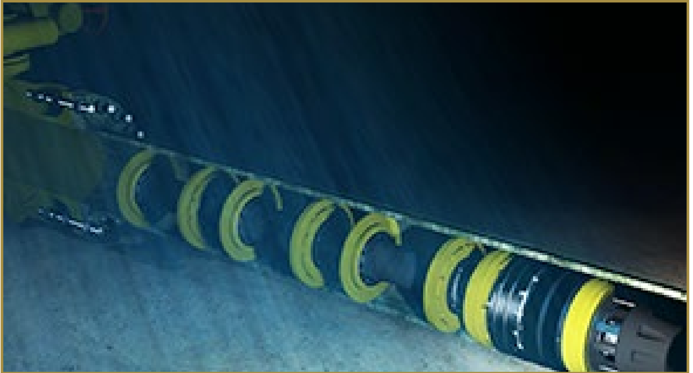
Tecno Plug™ isolates gas export pipeline to facilitate subsea metrology spool piece installation
