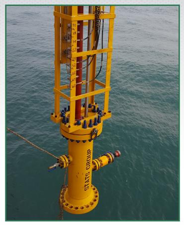
Following on from the success of significant subsea pipeline isolation and repair projects completed for the 28" Yacheng Pipeline in China and 8" subsea pipeline in the Gulf of Thailand, STATS Group (STATS) were selected for another major repair on the 14" subsea pipeline in East China Sea. STATS patented BISEP<sup>®</sup> was selected to provide leak-tight isolation of the pressurised pipeline whilst a damaged section of pipeline was cut and replaced.
