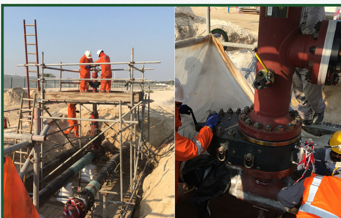
(Left) Hot tapping of existing pipeline to provide access for BISEP™ deployment. (Right) BISEP™ with integrated bypass during installation.
