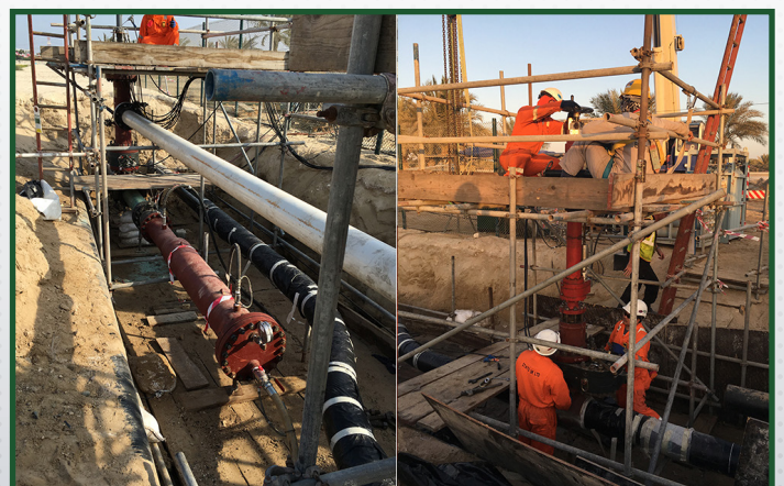
(Left) Temporary launcher attached to existing pipeline to allow recover of jet fuel, re-routed pipeline in place. (Right) Completion plug installation of welded fitting which will remain on the pipeline.
