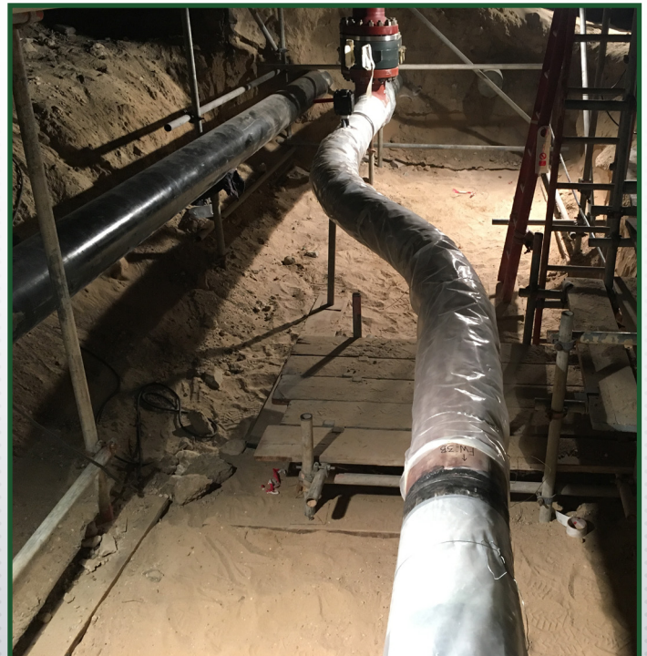
Pipe work re-routed
