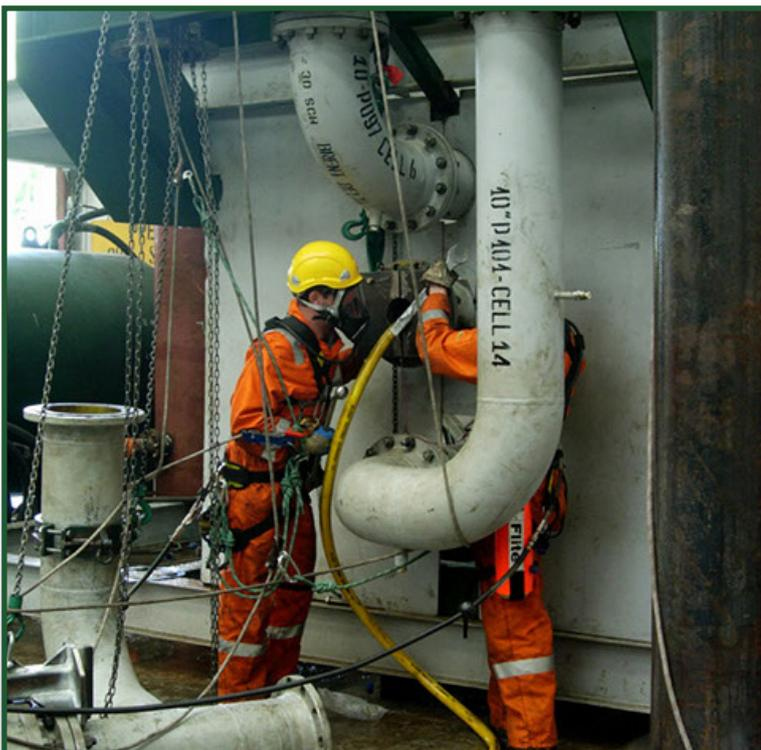
These slight, but critical differences in the platform piping required two distinctly different pigging disc and centraliser arrays to be developed for the Tecno Plugs™, the devil was in the detail.
