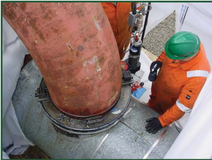
▲ 24" Header branch deconstruct, Gas Terminal, Scotland
