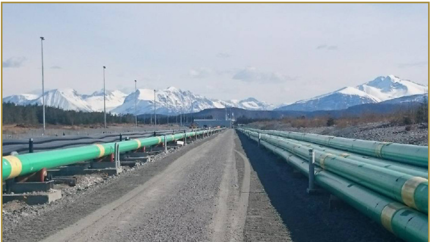
Spoolbase with welding station and pipe lay vessel in distance
