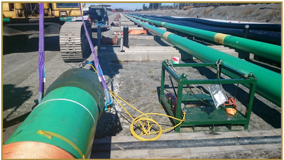
12" E-PEP installed to pipe spool
