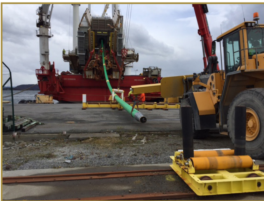
12" I-PEP installed in end of spool to allow reeling onto vessel
