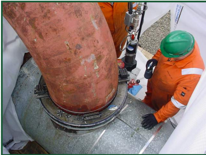
▲ 24" Header branch deconstruct, Gas Terminal, Scotland
