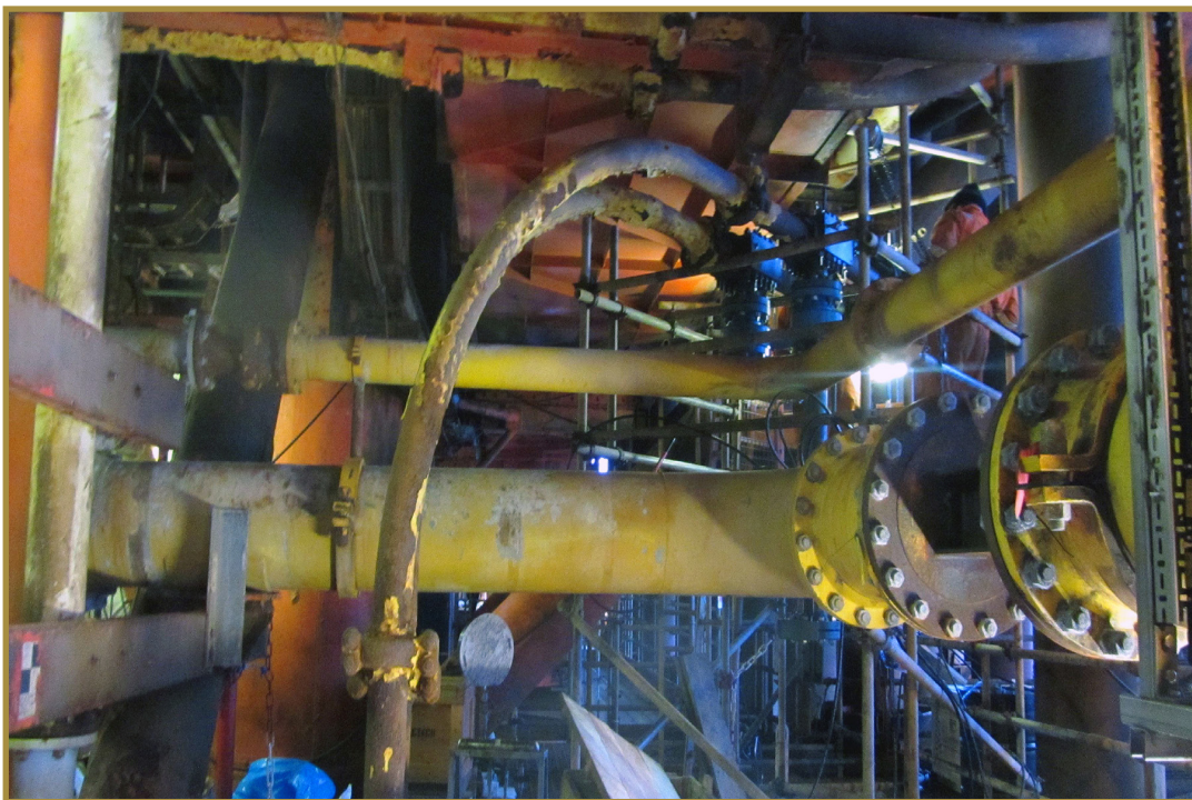
4" flowlines with mechanical tie-in clamps and BISEP™ installed
