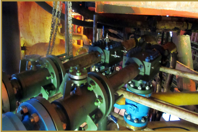
Flowlines isolated and mechanical connectors and valves installed
