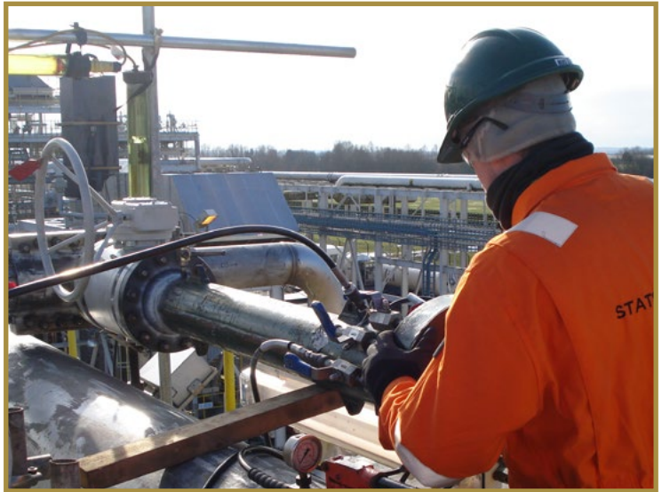
BISEP™ deployed providing double block and bleed isolation allowing valve changout
