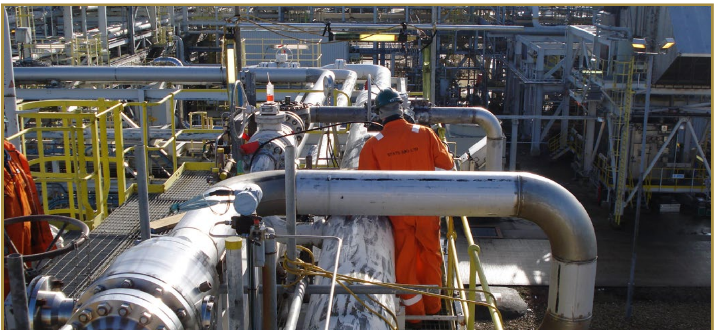
6" Hot tapping operation providing single penetration to deploy BISEP™
