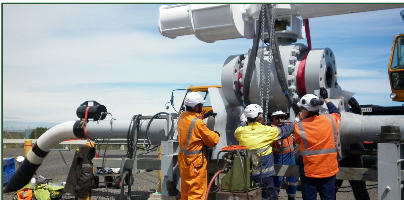
Remote Tecno Plug Isolating 72 bar gas pipeline to allow ESDV changeout
