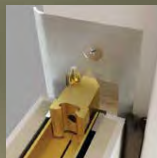
Angled shoulder on Bolt engages Roller Strike
