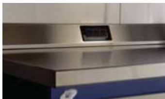
10 = power bar with 3 - 12A outlets for 15A circuit.
