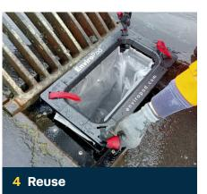
Reuse the Enviropod200 by placing securely back into the surrounding frame and seal, and close grate.
