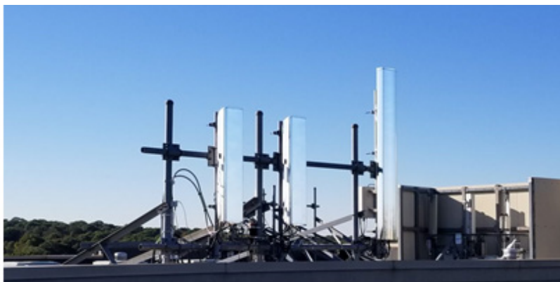
Figure 6: Antenna without Reflective Film (left) versus Antenna Applied with Reflective Film (right)
