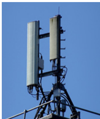
Figure 6: Antenna without Reflective Film (left) versus Antenna Applied with Reflective Film (right)
