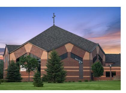
The key selling feature was the interlocking nature of DECRA's direct to deck products. During the installation process, the clip-lock at the nose of one panel and the clip-lock at the back of another are interlocked and screwed down. Likewise, there is a side-lap locking mechanism contributing to the interlocking nature of the product. This installation process allows DECRA products to be warranted against winds up to 120 mph.
