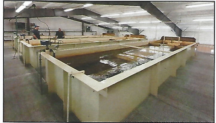
Figure 4 The plant repaired and painted the tanks during the repair-upgrade process.
