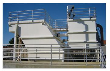
WesTech inclined **SuperSettler™ Plate Packs** are designed for installation on support beams in rectangular concrete basins. After the inlet flow enters the basin, it is directed to inlet ports on the side of each inclined plate. Outlet launders at the top of the plate packs collect the clarified water as solids settle out on the plates and then the basin floor. The ZICKERT Shark™ is an ideal sludge removal device for SuperSettler™ basins.
