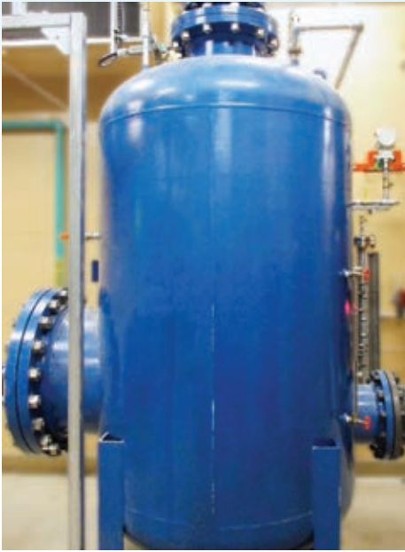
WesTech provided pressurization vessels for the plant's new unit and four upgraded units.
