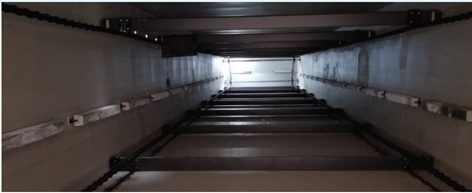
The oil/water separators are constructed of corrosion-resistant materials inside and out.
