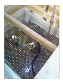
Webster City moved forward with installing the WesTech MULTIWASH backwash enhancement. The plant's filter runs are now in excess of 100 hours. MULTIWASH also provides a vigorous backwash which efficiently cleans the filter media, eliminating the plant's concern that a water-only backwash would not adequately clean the media. MULTIWASH troughs have low-profile media retaining baffles to help with the plant's media retention.
