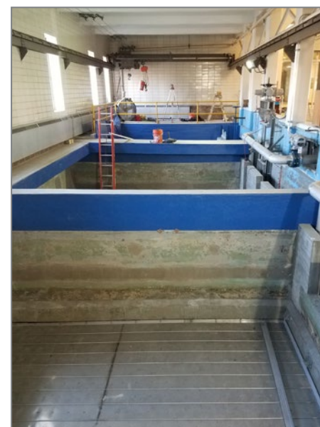
Completed LAZERFLO underdrain
