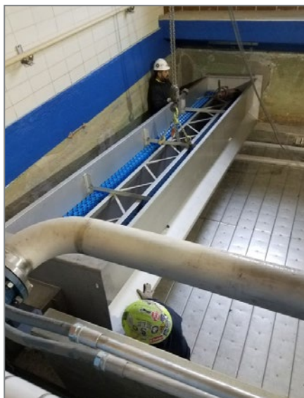
Installing MULTIWASH with LAZERFLO underdrain system
