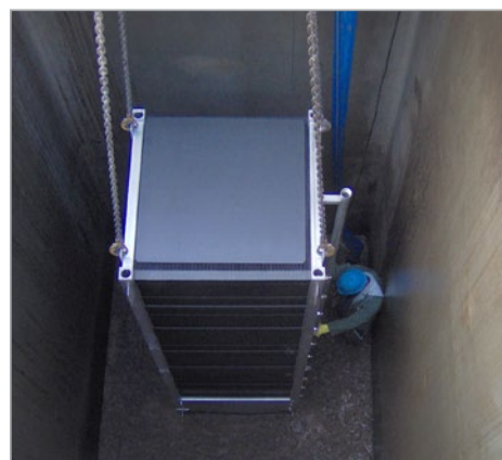
ClearLogic® MBR Installation
