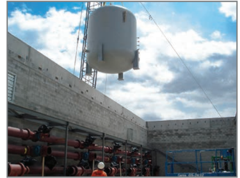
Installation of Vertical Pressure Filters for BIOBROx® Process
