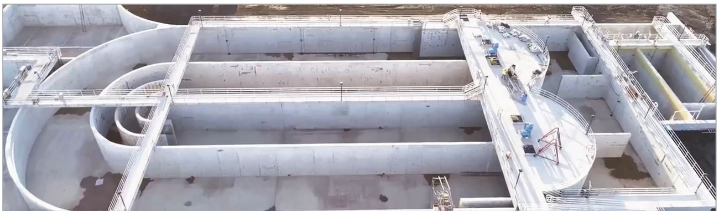
Under Construction: The Wakarusa WWTP OxyStream Oxidation Ditch
