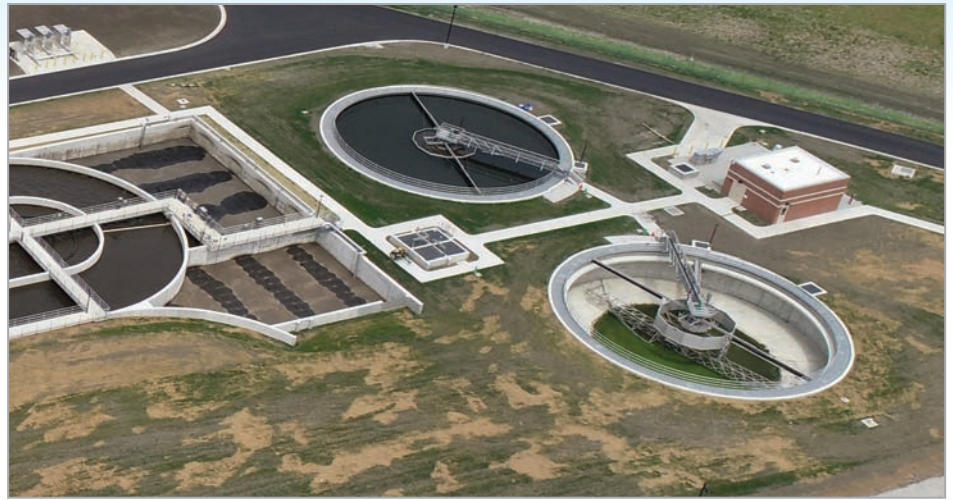
Two COP Clarifiers Ensure the Capacity for Future Growth
