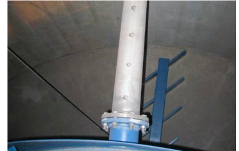
Weir and Rake Arm
