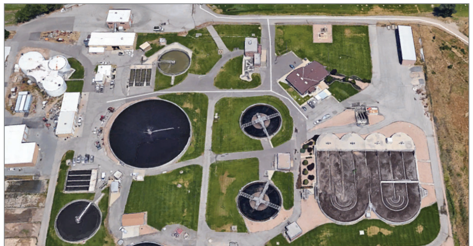
Aerial view of the Central Davis Sewer District WWTP
