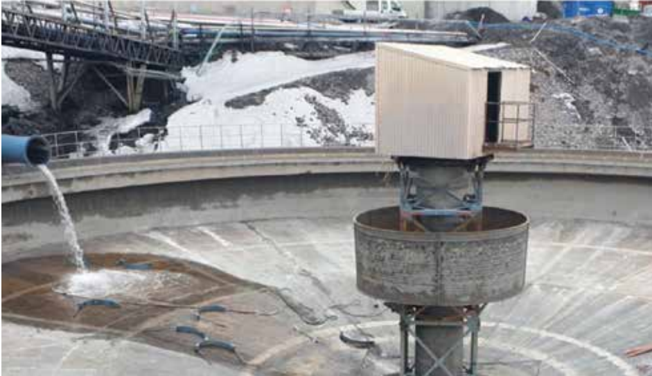
Vinab began by removing all equipment from the thickener basins.
