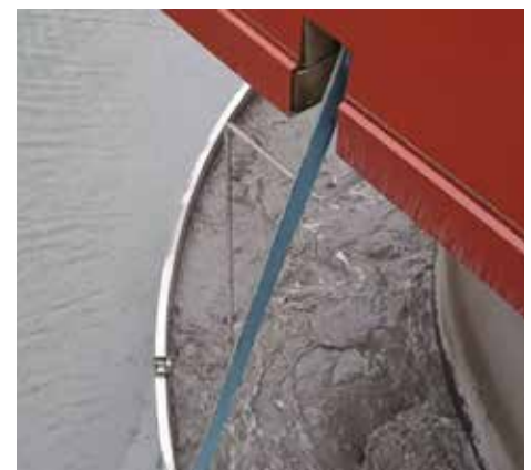
Adjusting the EvenFlo's ports for the actual flow rate of 3,700 m 3 /h further improved effluent clarity.
