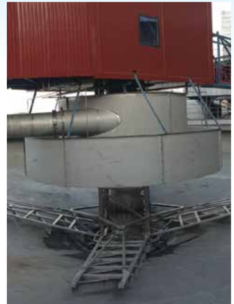
The EvenFlo uses a two-stage design that prevents short-circuiting and reduces chemical usage.
