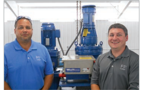
Paul Nail, General Manager (L) and Brandon Light, (R) Plant Manager, Fort Payne Water District
