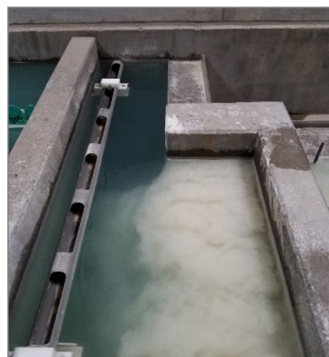
Picture of solids in properly operating clarifier
