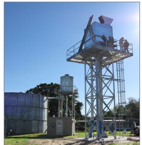
Existing and New Forced Draft Aerators
